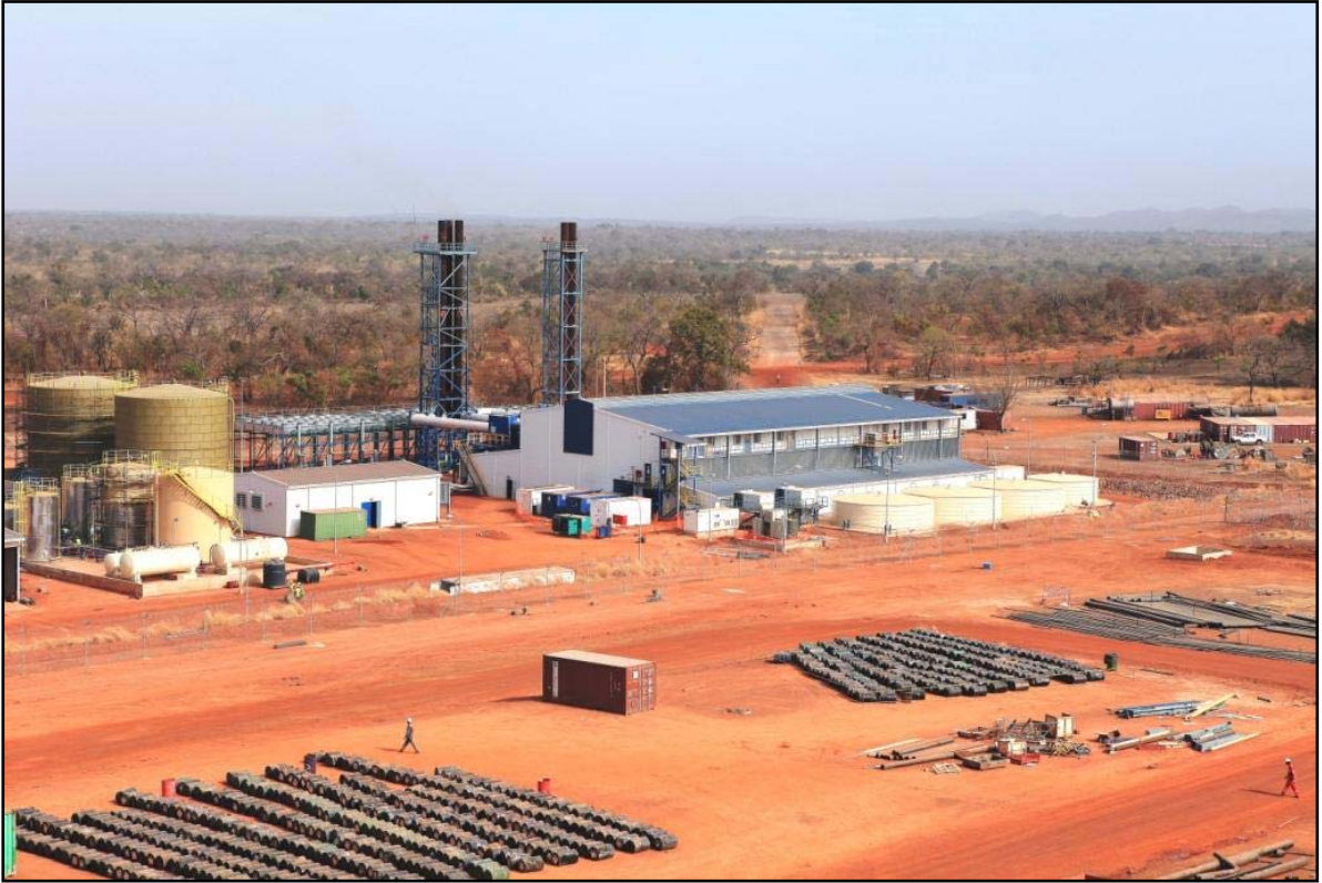
Power Station - 30MW
