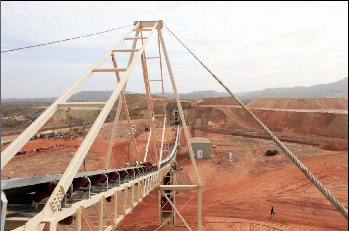
Crushing circuit with conveyor belt stacker and showing ROM pad in the background
