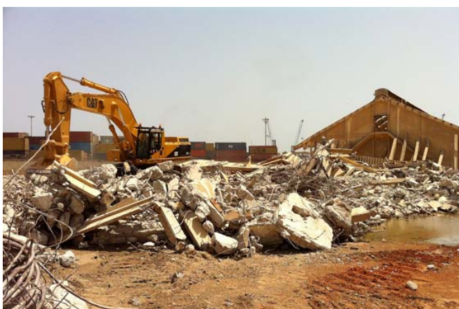
Demolition of existing building on 30,000m 2 port site
