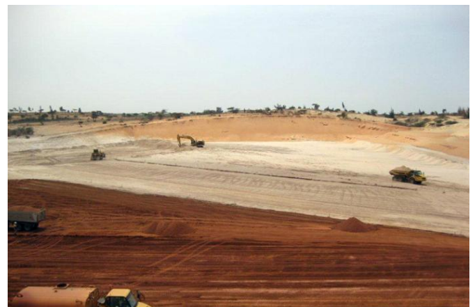
Excavation of initial dredge pond
