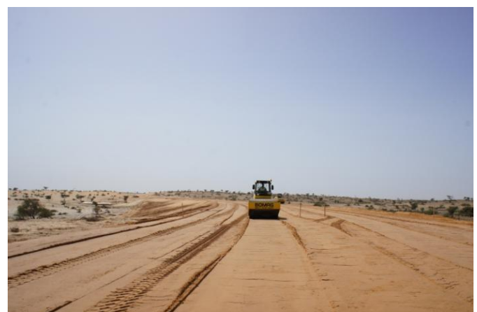
Earthworks on rail corridor between MSP and existing rail
