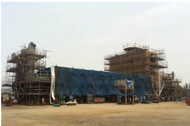
Dredge taking shape in Thailand
