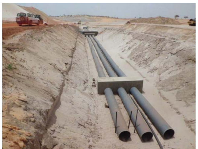
Pipe installation linking dam and initial dredge site
