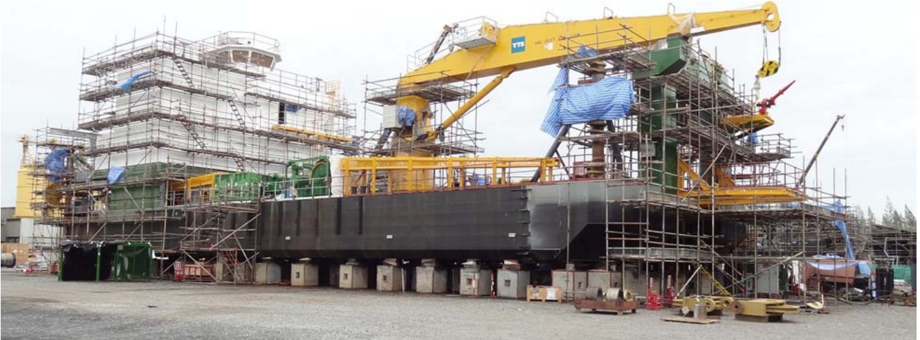
Dredge build in Thailand now nearly 90% complete
