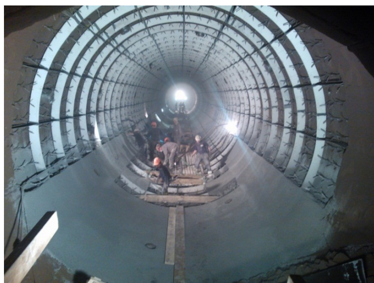
Casting of the new refractory lining in the pre-reduction rotary kiln
