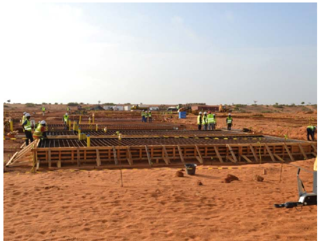
Engine slabs for power station being laid
