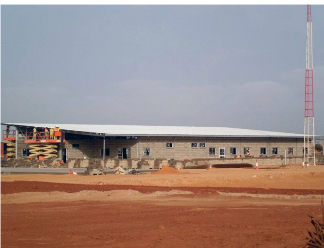
Construction of administration building at MSP
