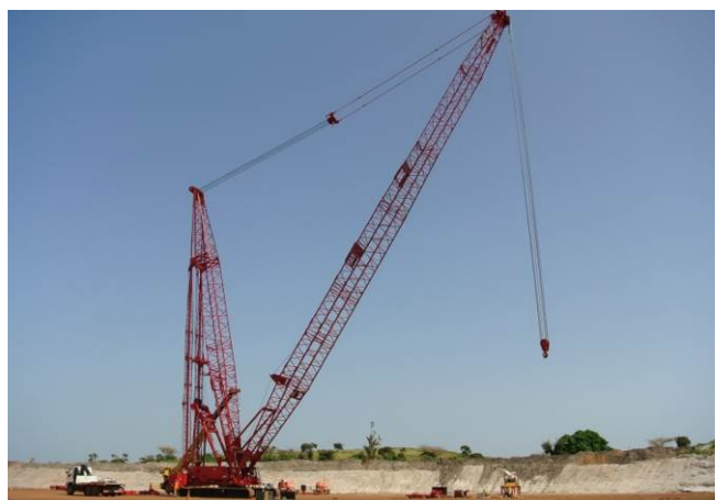
500 tonne crane ready for wet concentrator construction
