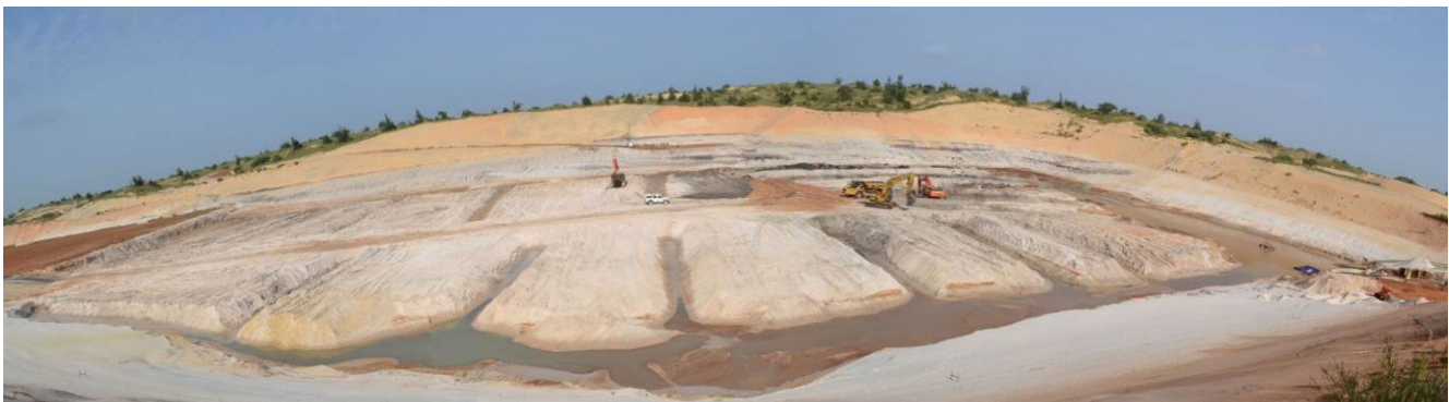
Excavation at dredge pond start-up area reaches water table
