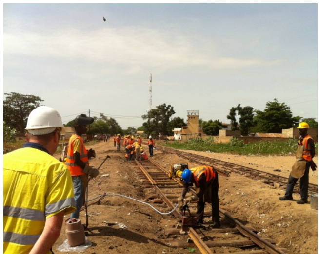
Refurbishment of existing rail
