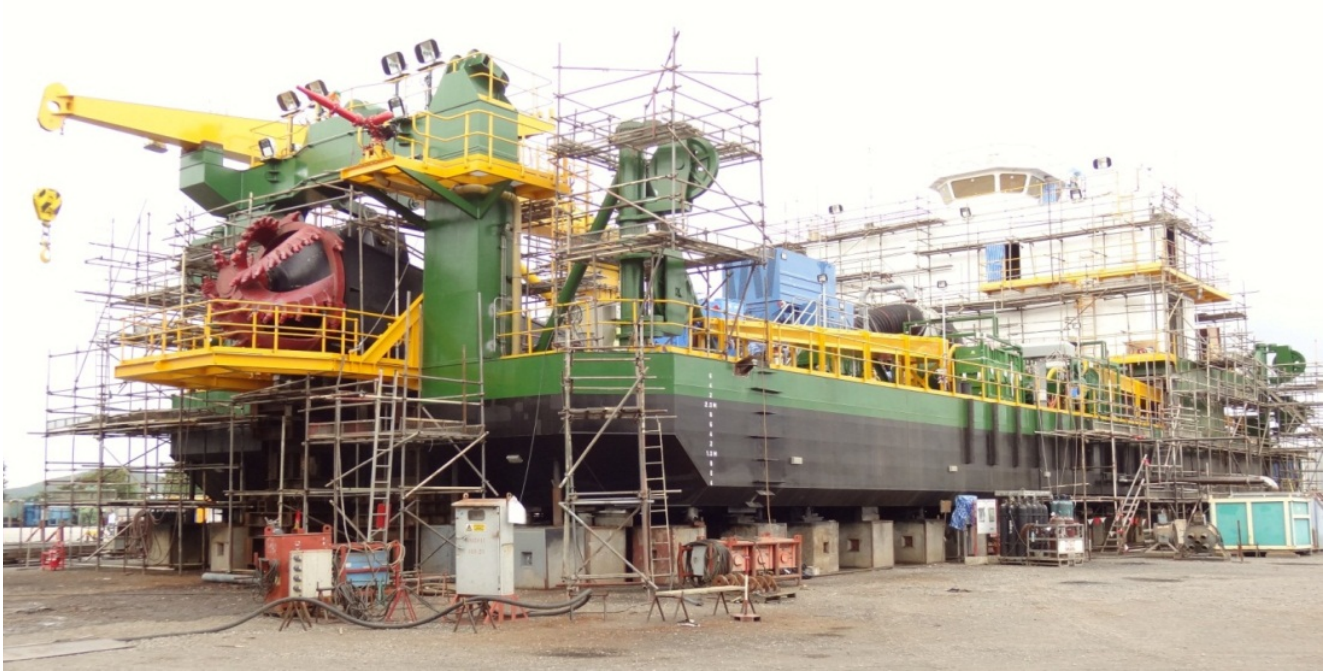
The dredge fully assembled in Thailand, prior to being disassembled and packed for shipment to site
