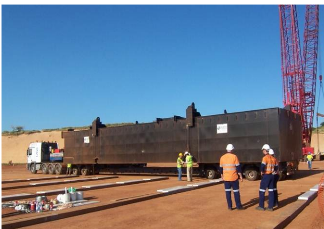
The first of 41 floating plant pontoons arrive on site
