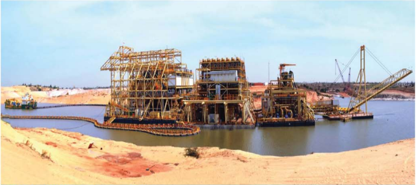
Dredge and Wet Concentrator Plant (WCP)
