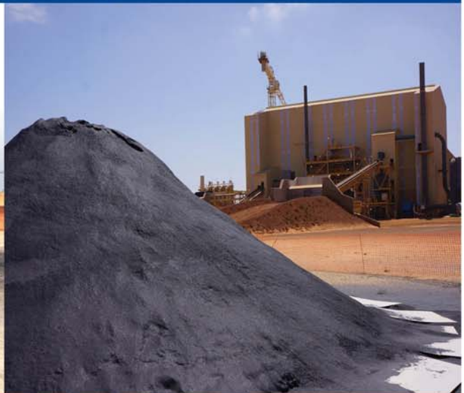
View of the Dry Mill at the MSP
