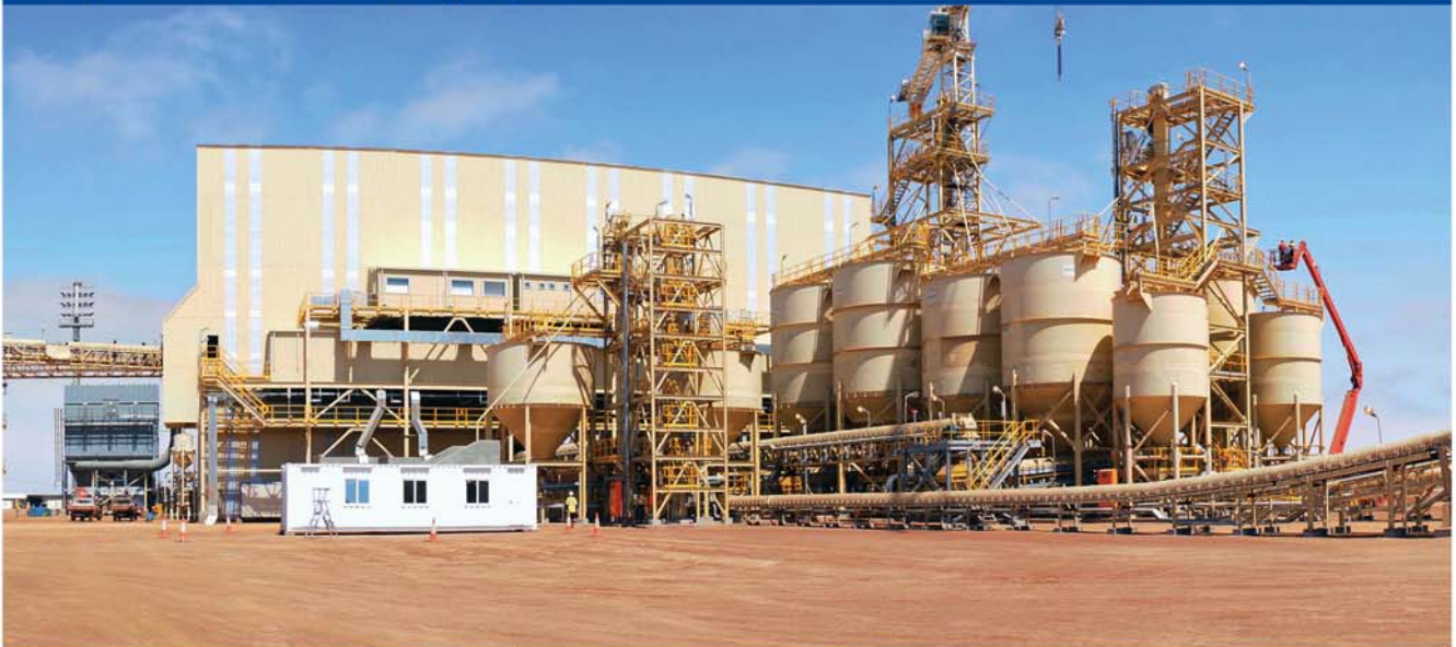
Dry Mill at the Mineral Separation Plant (MSP) with zircon and rutile storage
