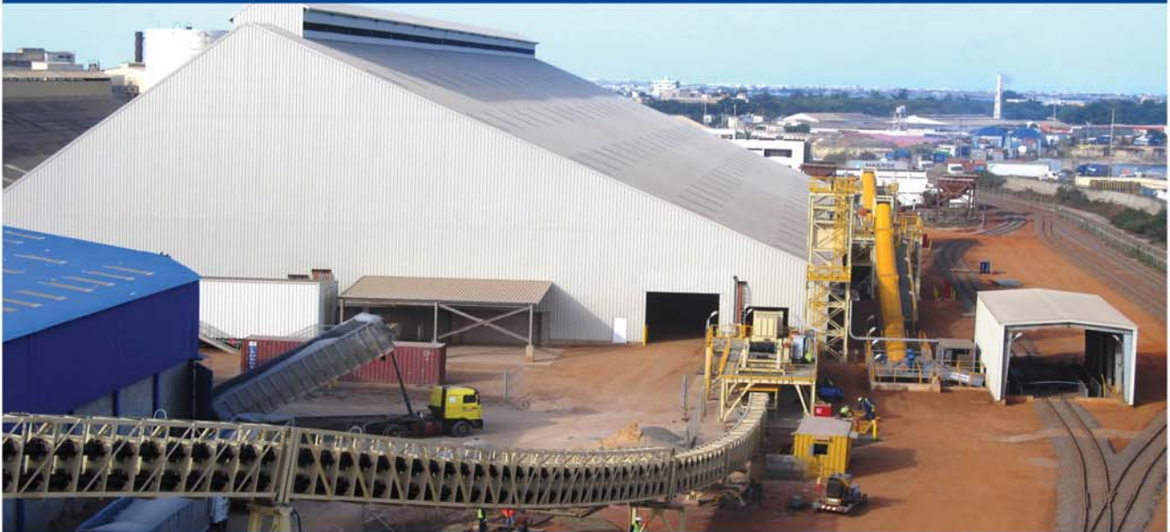
Storage and conveyor facilities at Dakar port
