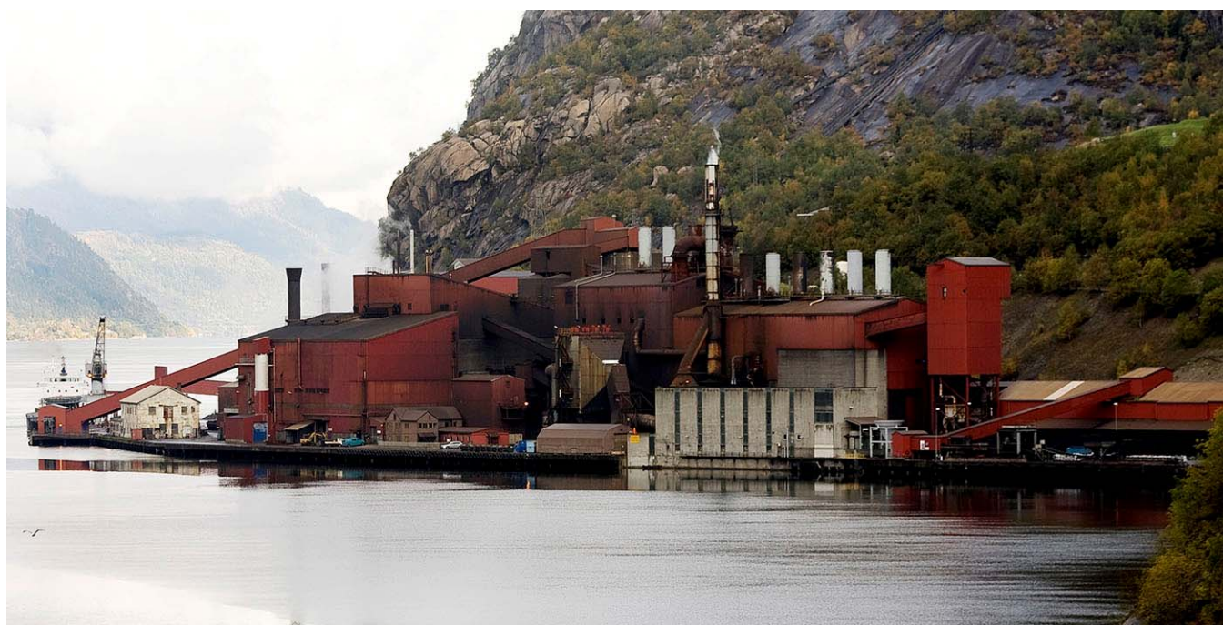
Tyssedal ilmenite upgrading facility, Norway
